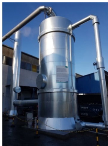
Figure 2. Working CTBB during tests of bio-purification of air in real conditions of Enduser. Source: own elaboration
